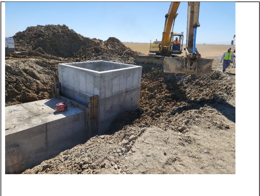
Pump sump and box culvert.
