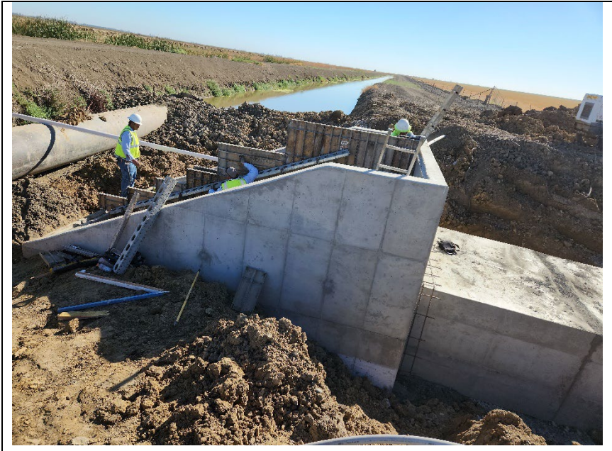
Inlet structure and box culvert.
